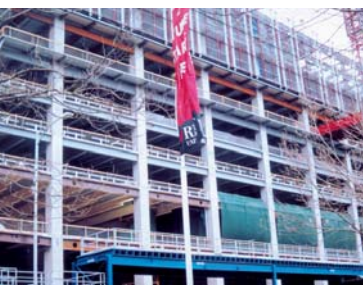
The Queen Victoria Building (QVB) Melbourne is a steel-frame building and is a good example of increased usage of steel in a multi-level building.
