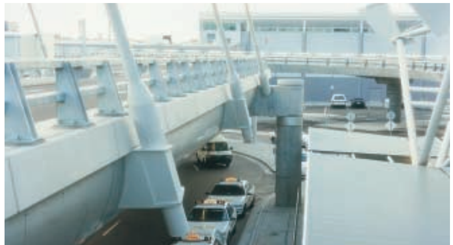
External cable connections kept deck width to a minimum.
