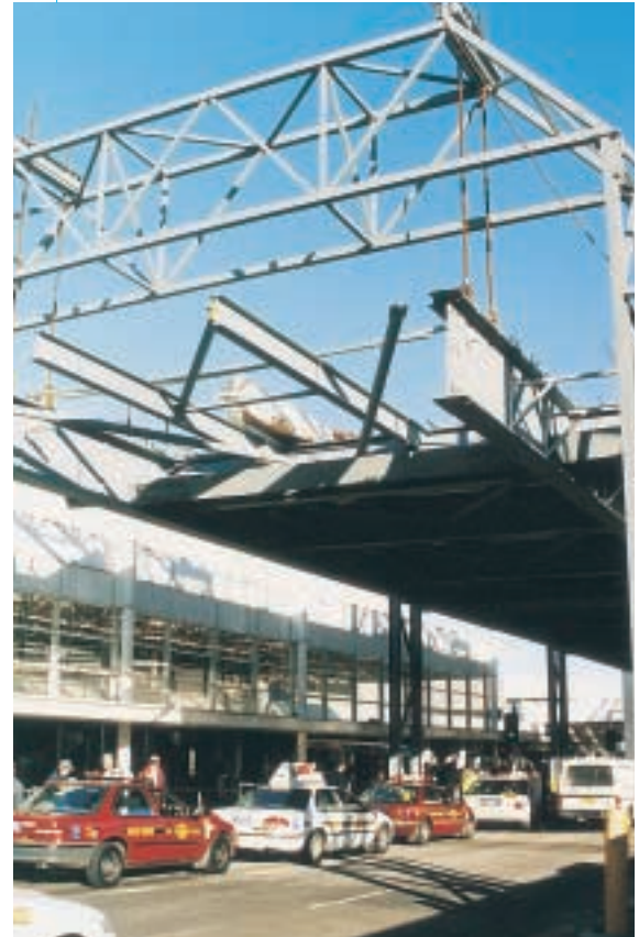
Construction of the elevated roadway was achieved with minimal disruption to traffic below.
