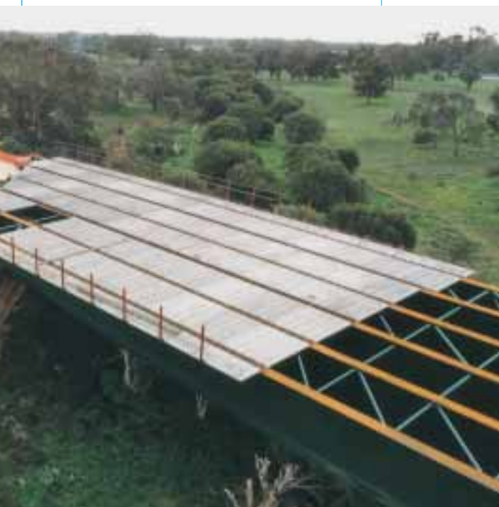
Opposite, top: The 56 metre span leaves an Aboriginal sacred site undisturbed.
